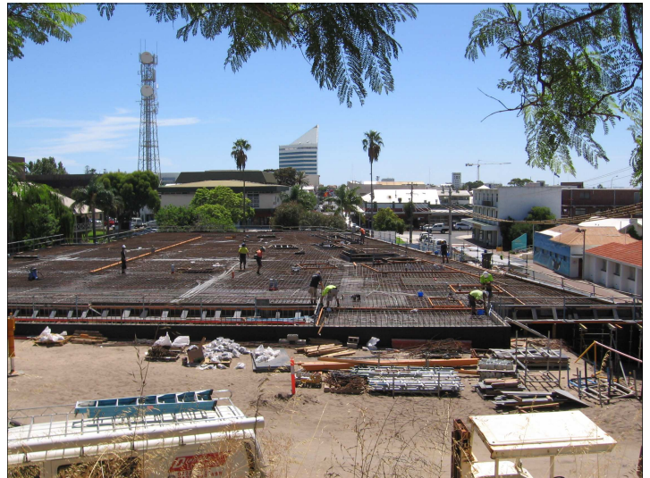
Formwork ready for the big pour, 11 March 2008
