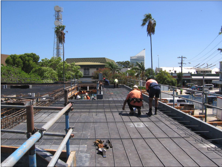
Preparing formwork and steel fixing for Library floor, mid-February 2008
