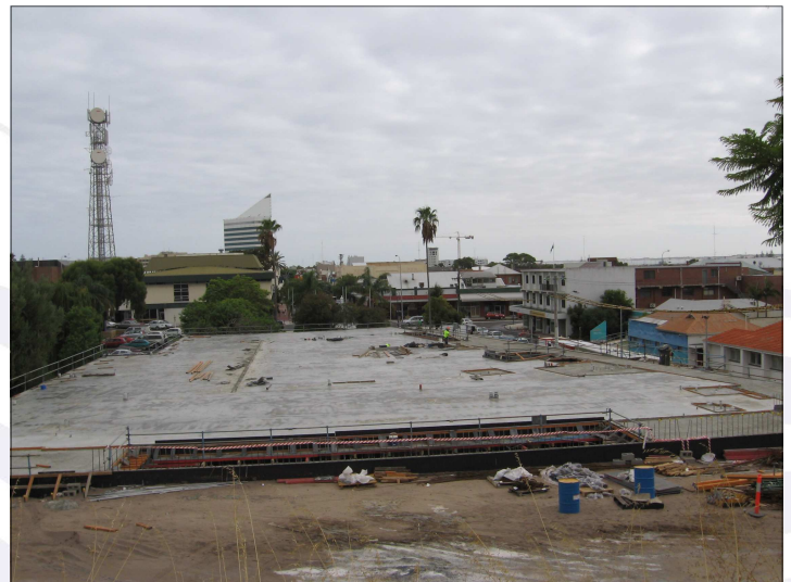
The completed Library floor, 13 March 2008
